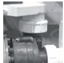
Slice Valve and Pump Union
