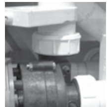
Slice Valve and Pump Union
