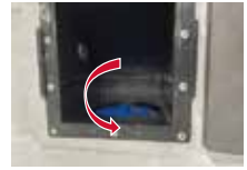
Turn Filter Counter-clockwise to Remove
