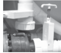
Slice Valve and Pump Union
